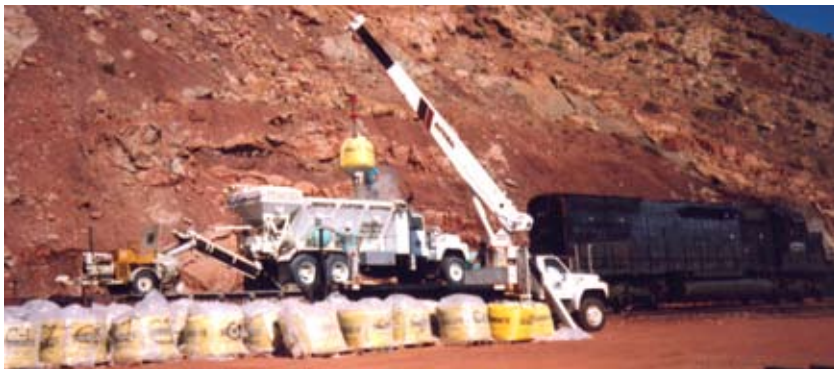
Shotcrete (approx. 400 cu. yards) utilized on retention pond for South Canyon Landfill. --- Glenwood Springs, CO
