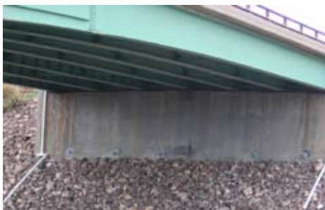
Soil nailed overpass abatement.
