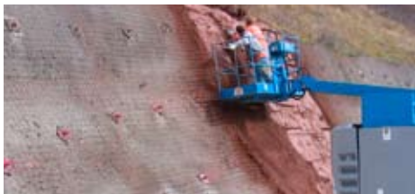
Soil nailed wall with carved shotcrete.
