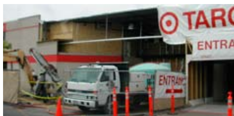
Installing micropiles on Target Store expansion - Grand Junction, CO
