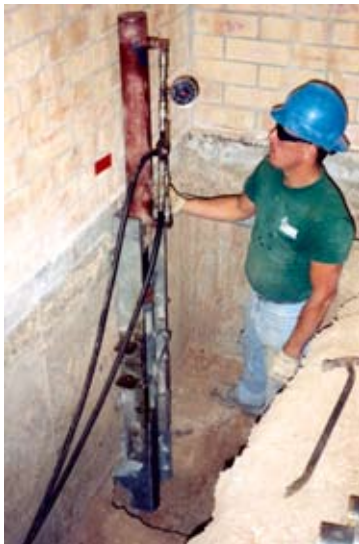
Underpinning at Northwest Community College. ---Rangely, CO
